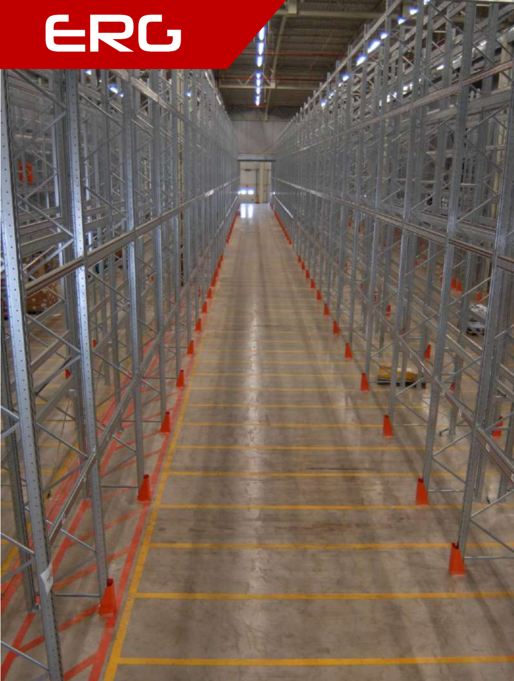
High view of pallet racking system.
