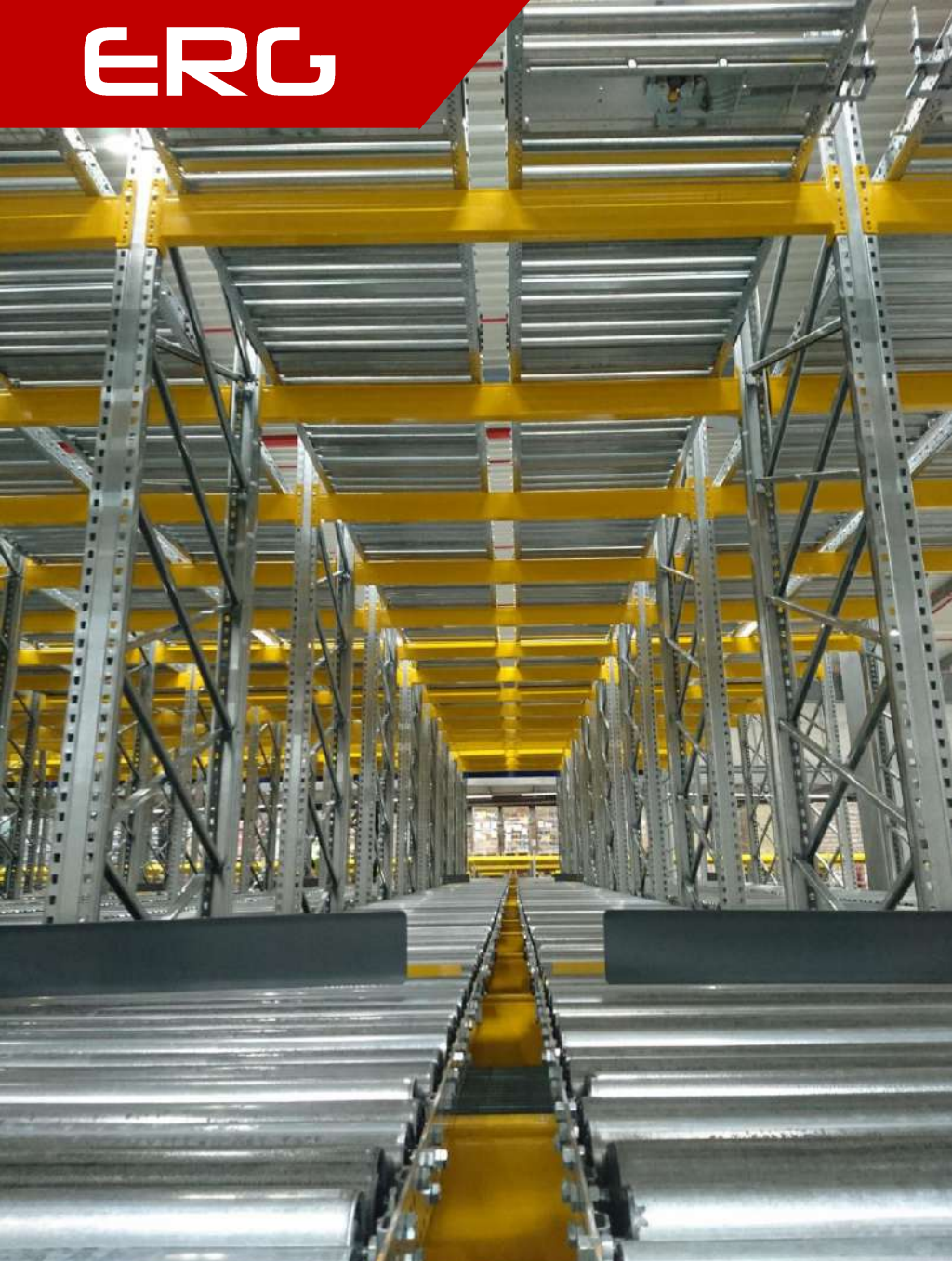
Detail of tunnel with rollers FIFO.
