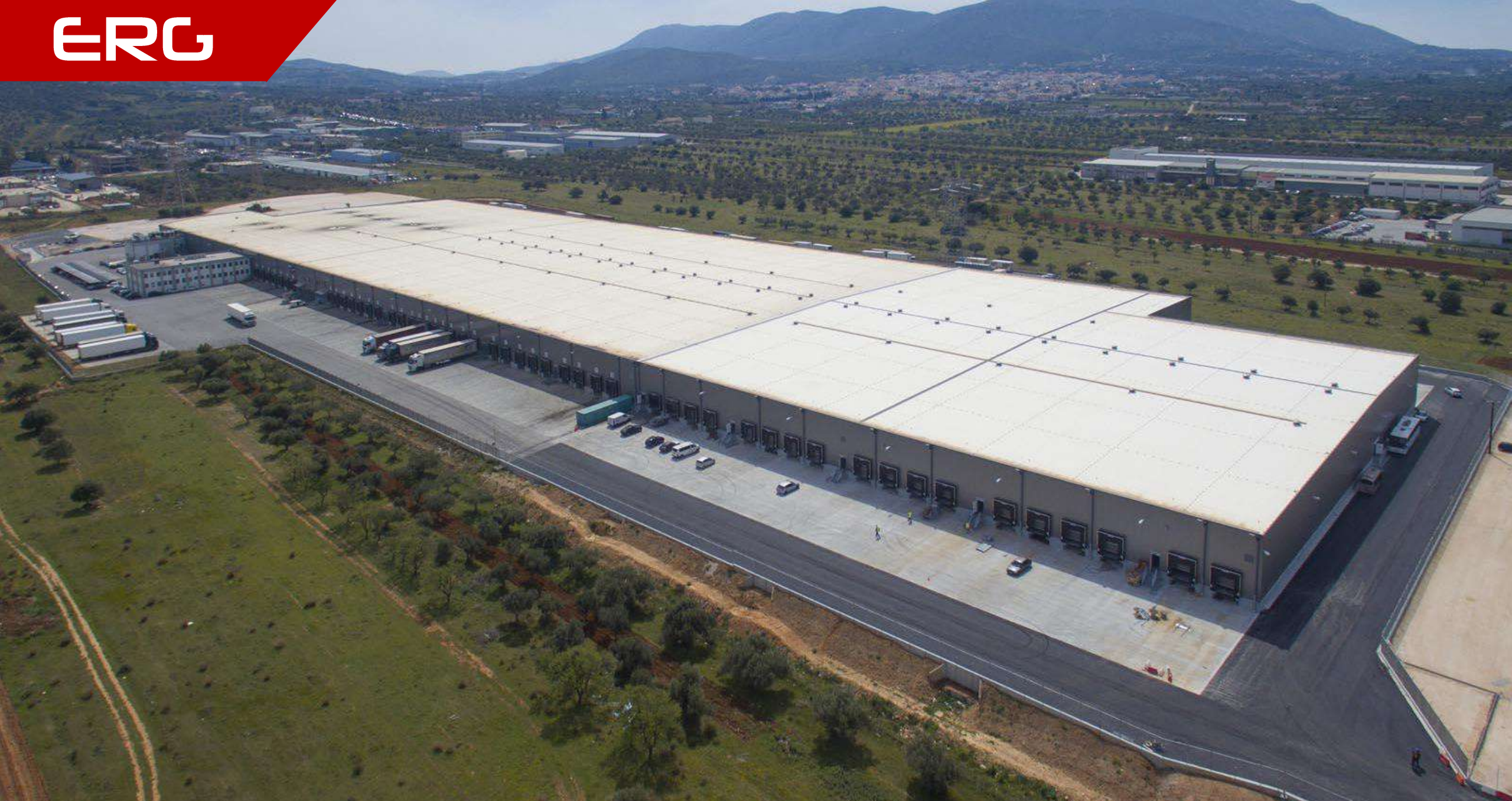
Aerial view of the warehouse.
