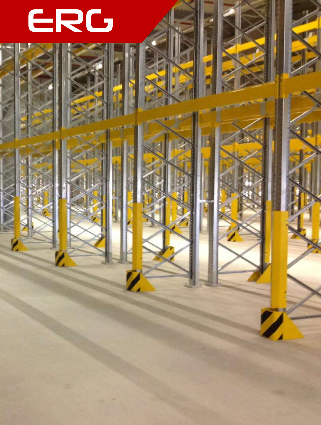
View of pallet racking system.
