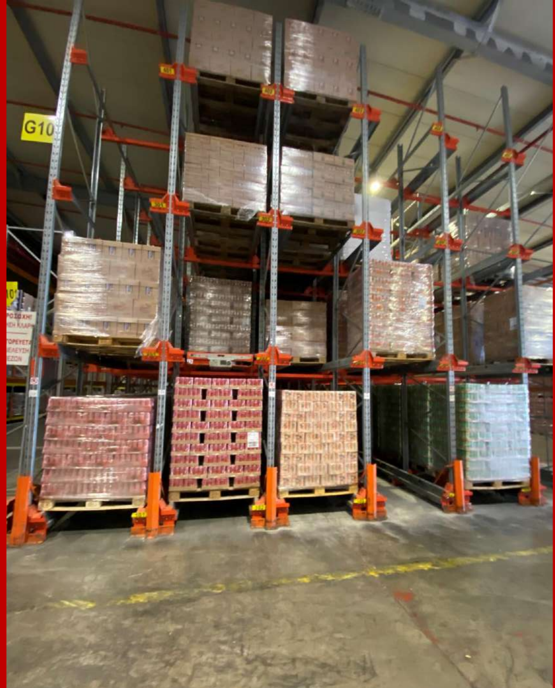
Front view of satellite block.
