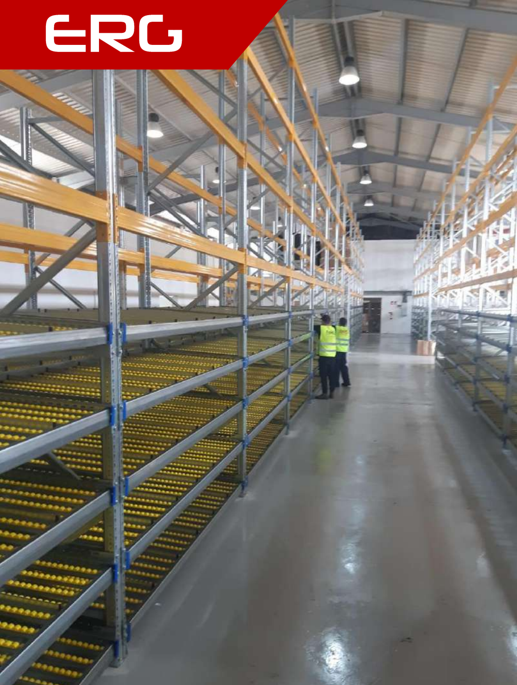
Installation phase of carton live storage.
