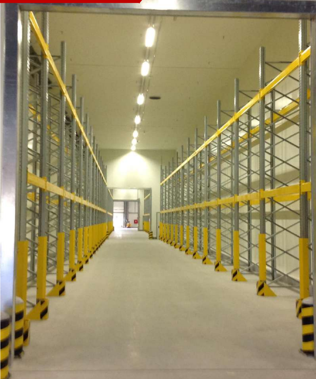
View of pallet racking system.
