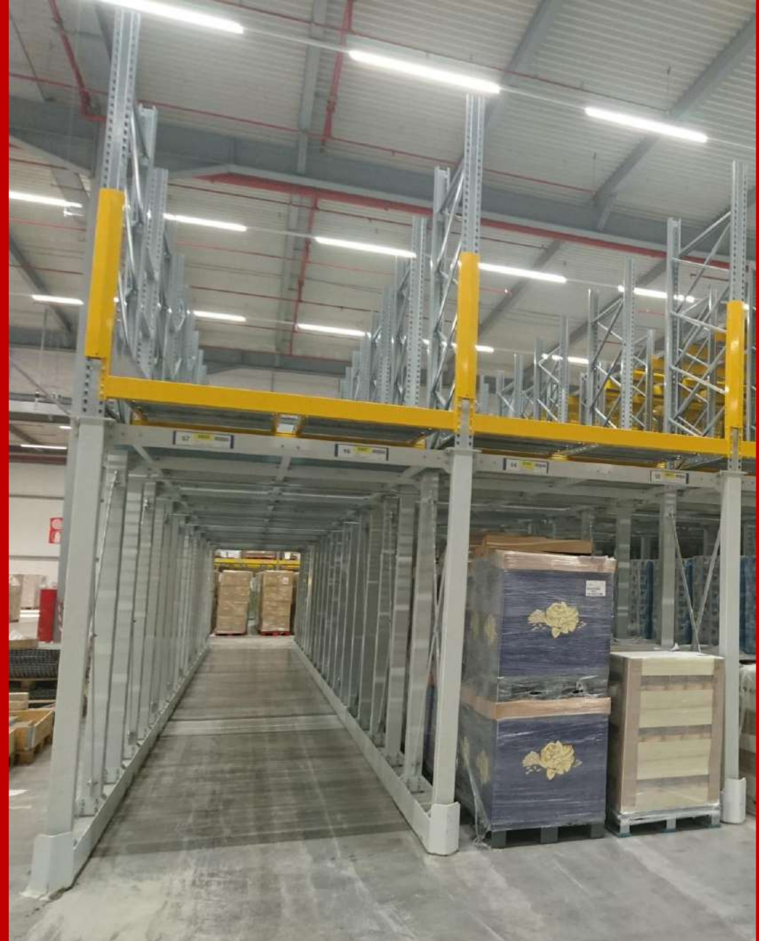
View of ground tunnels (in progress).
