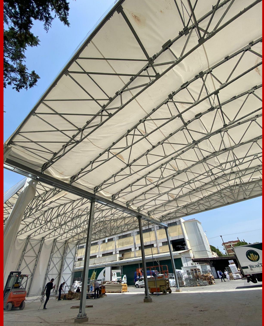
Steel structure of the building with the shared columns.
