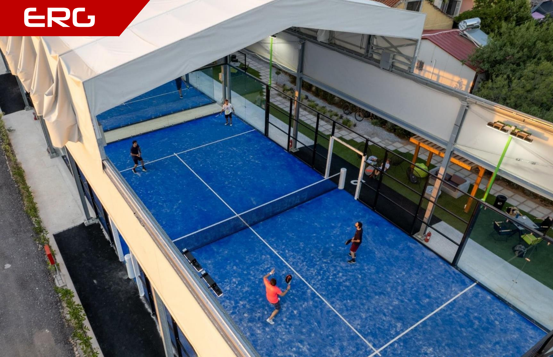
Aerial view of the entire structure.
