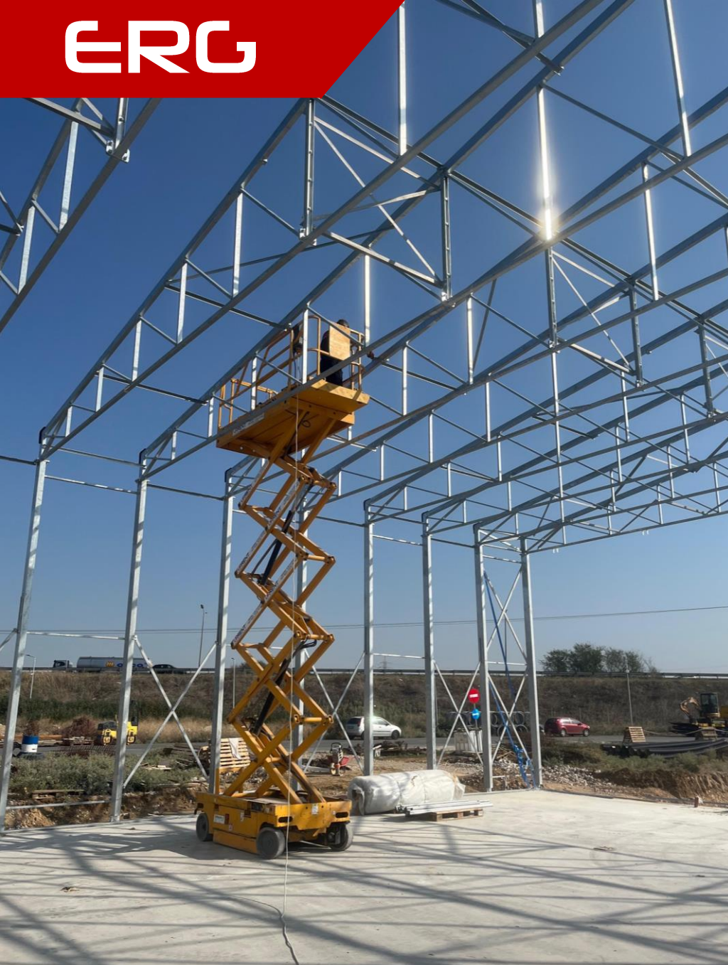
Steel structure assembly (Under construction).
