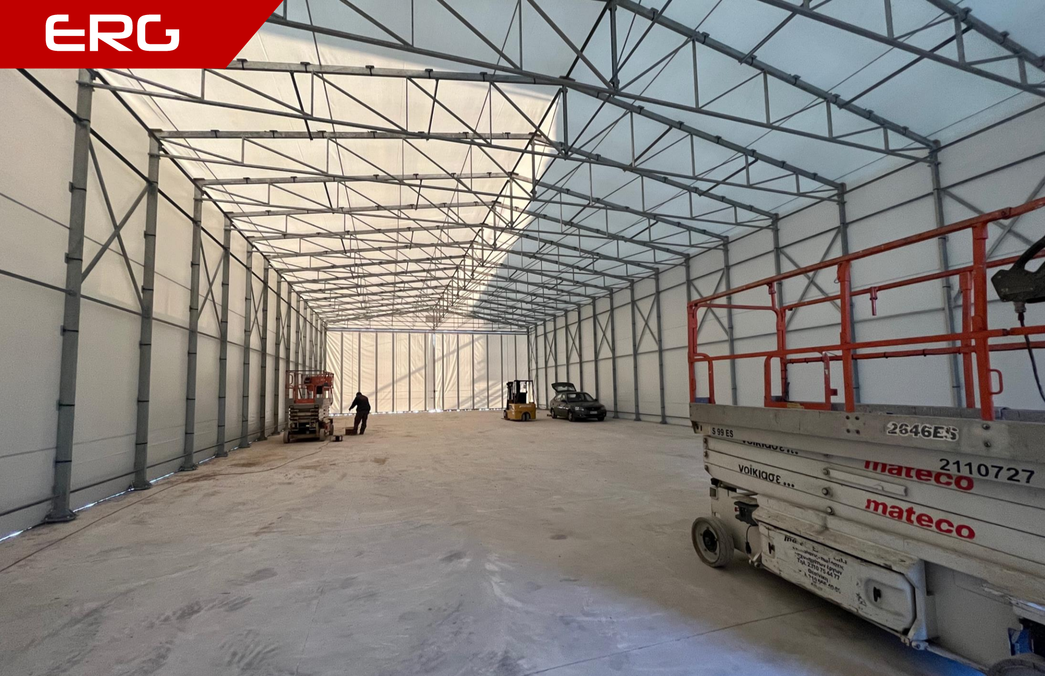
Interior of the fixed building.
