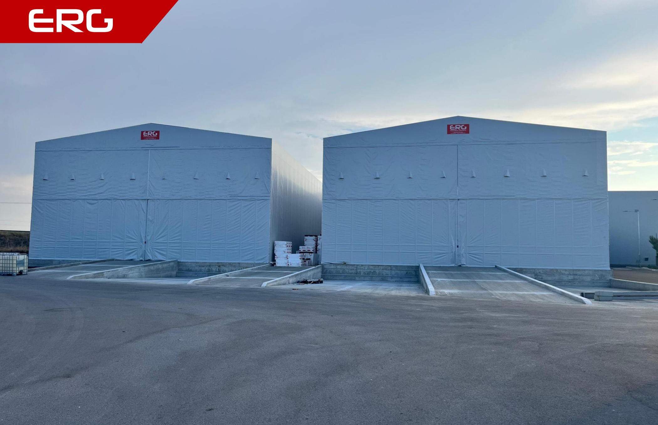
Exterior view of the buildings with sliding curtains closed (in use).
