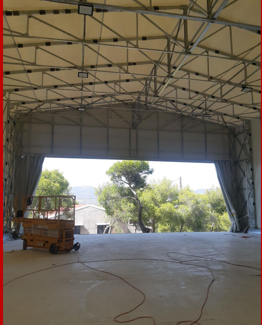
Interior of the building. (Under construction)
