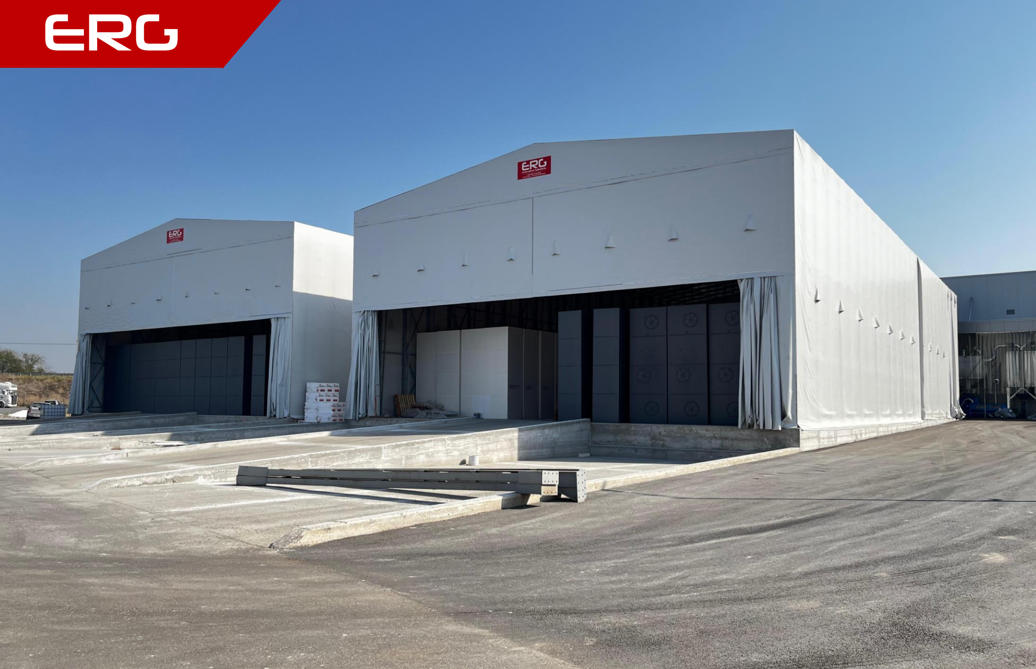
Exterior view of the buildings with PVC covers on (in use).
