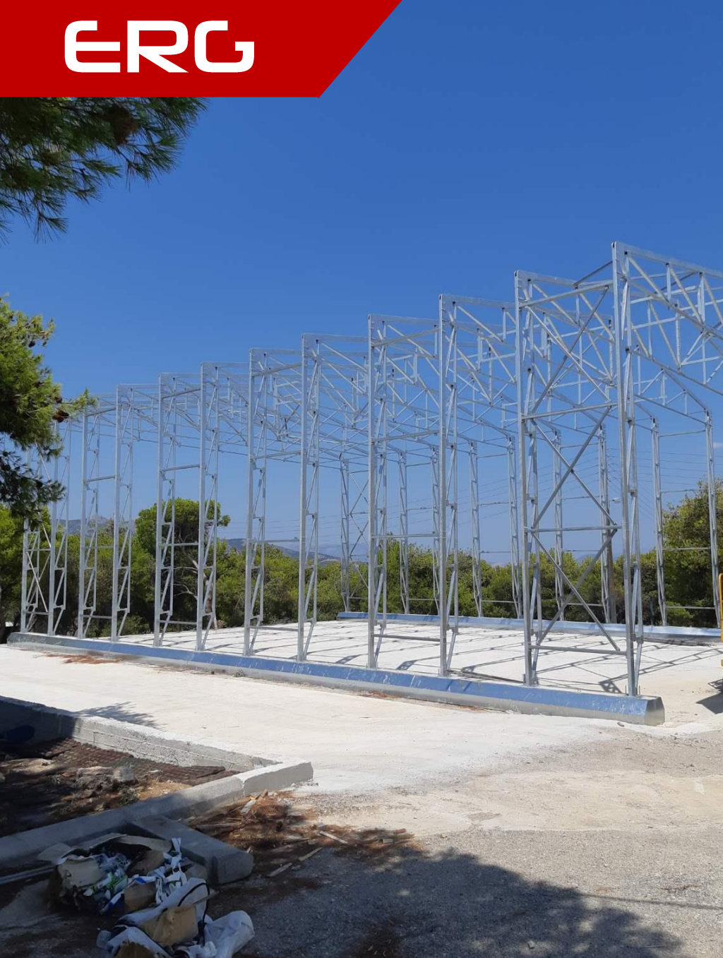
Steel structure frame.
