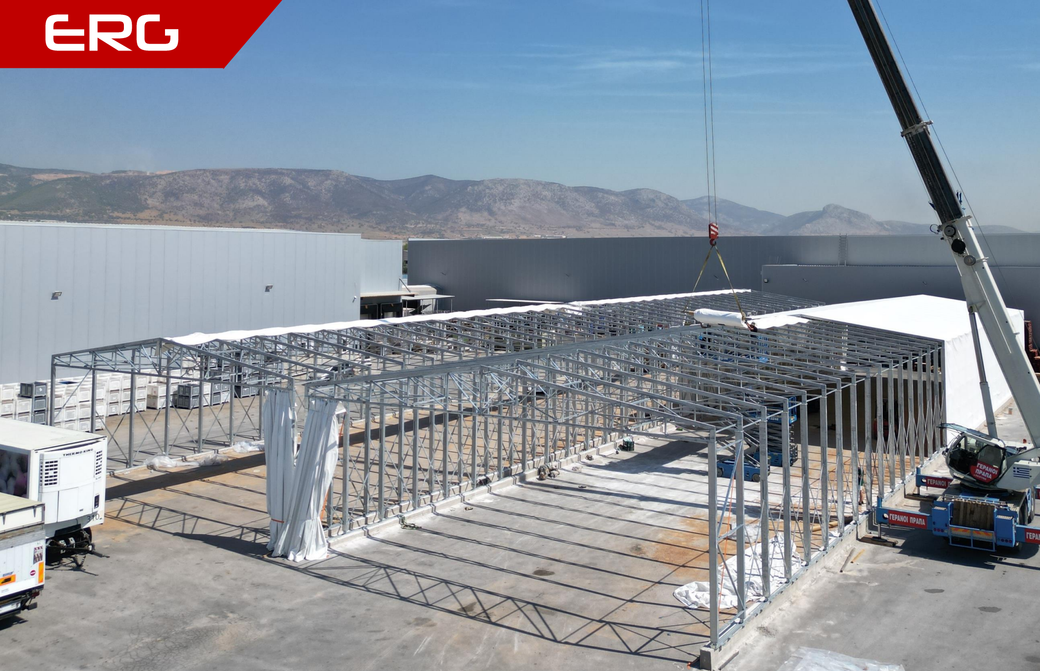
Steel structure frames (Under construction).
