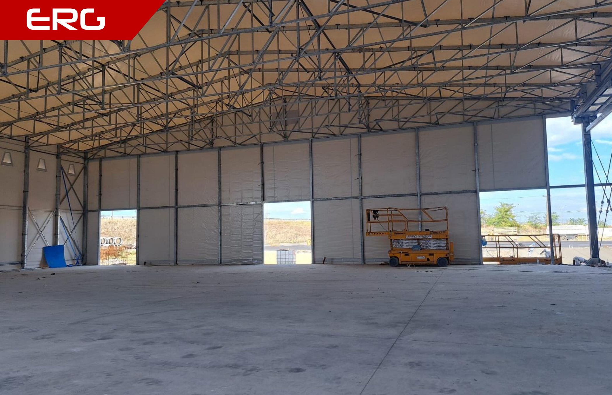
Interior view of the buildings (Under construction).
