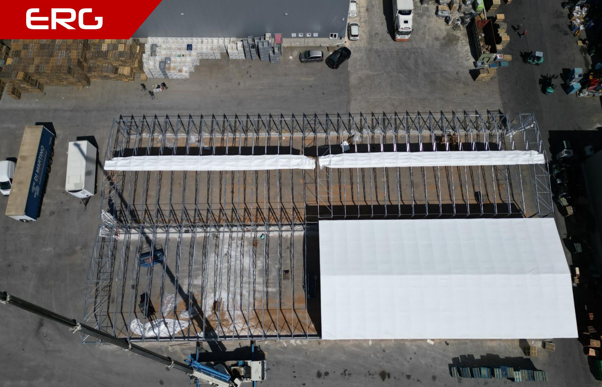
Steel structure frames (Under construction).
