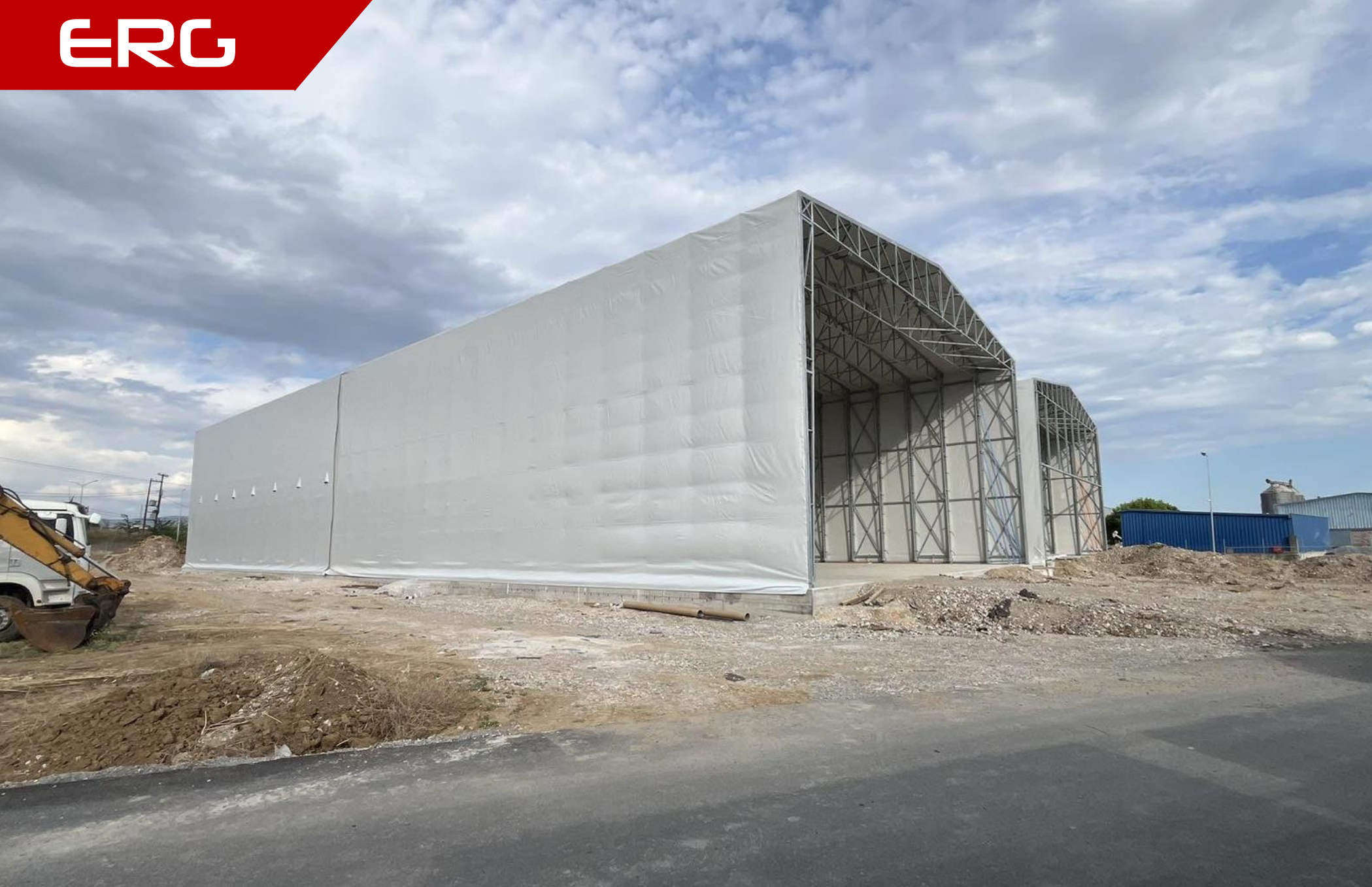
Exterior view of the buildings with PVC covers on (Under construction).
