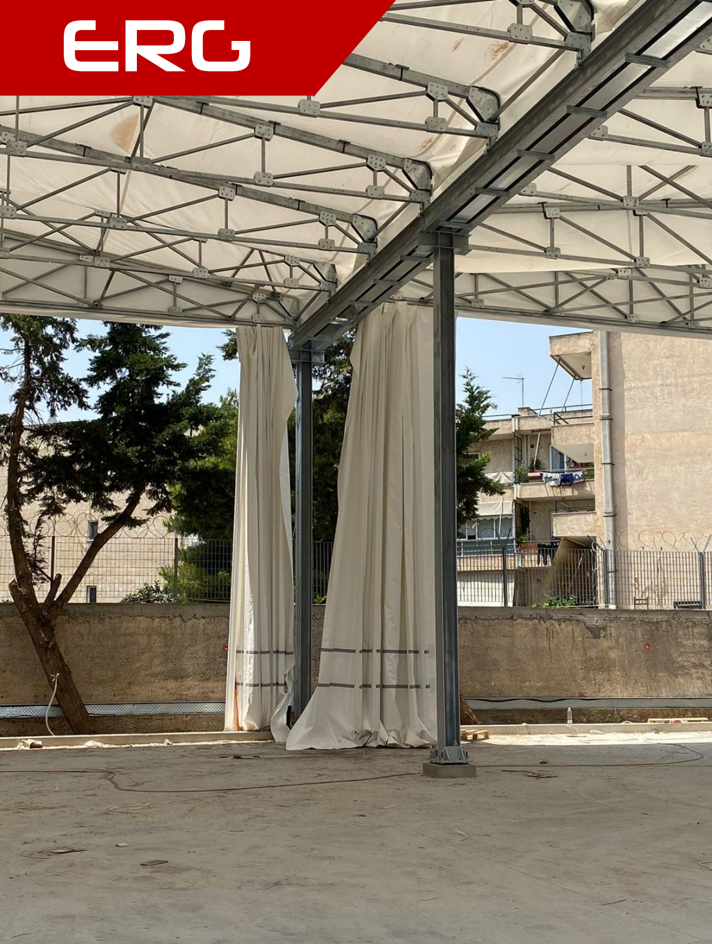
Interior of the building (Under construction).
