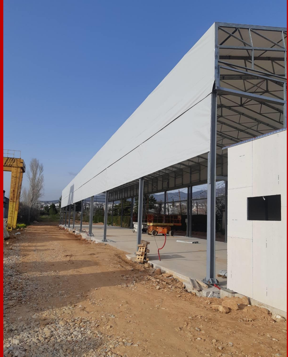
Exterior of the hangar with PVC cover on. (Under construction)
