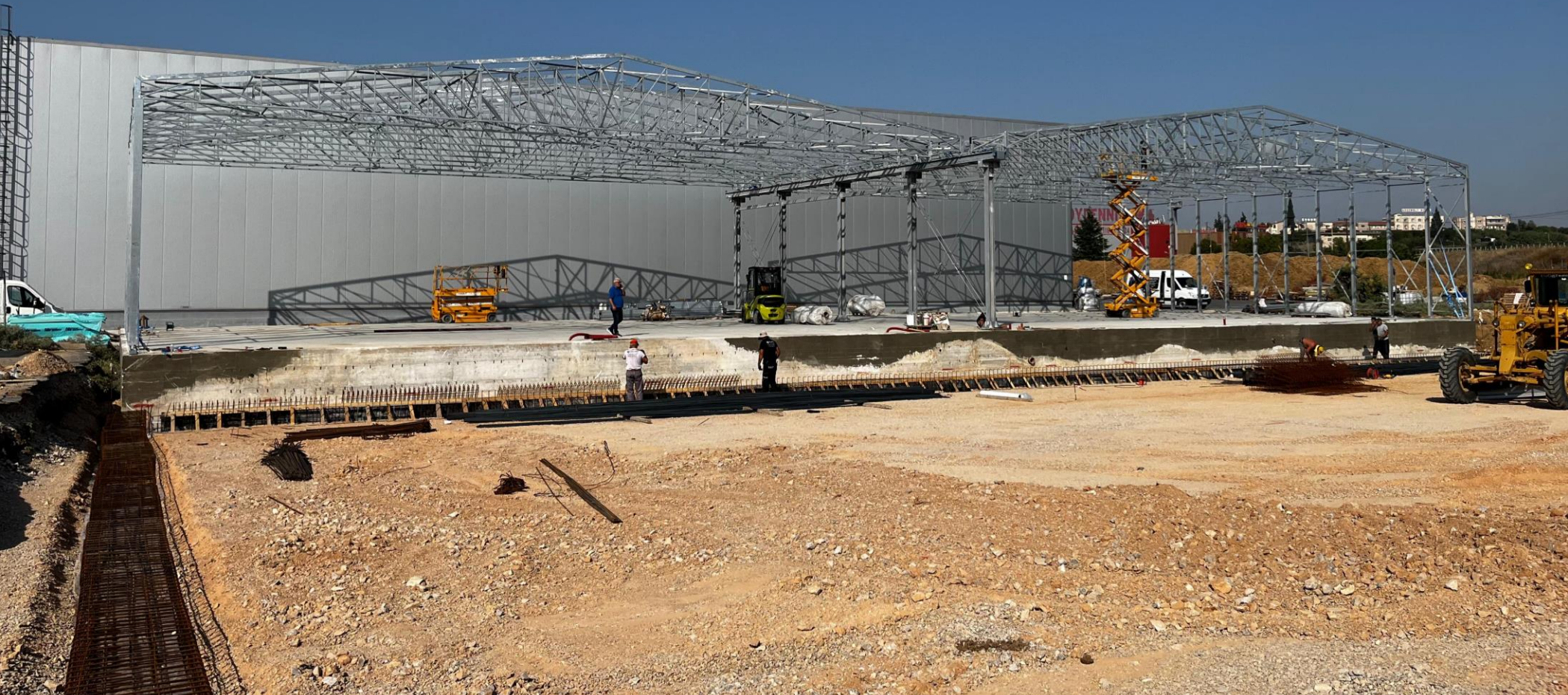
Steel structure frame (Under construction).
