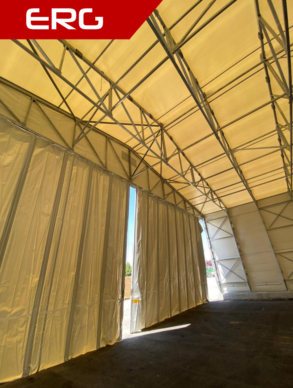
Interior of the tunnel.
