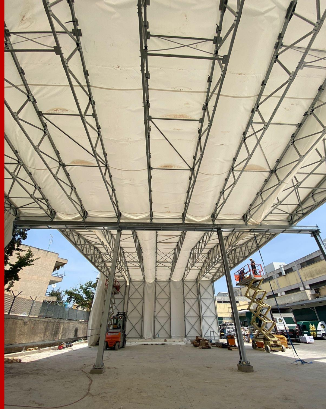
Interior of the building (Under construction).
