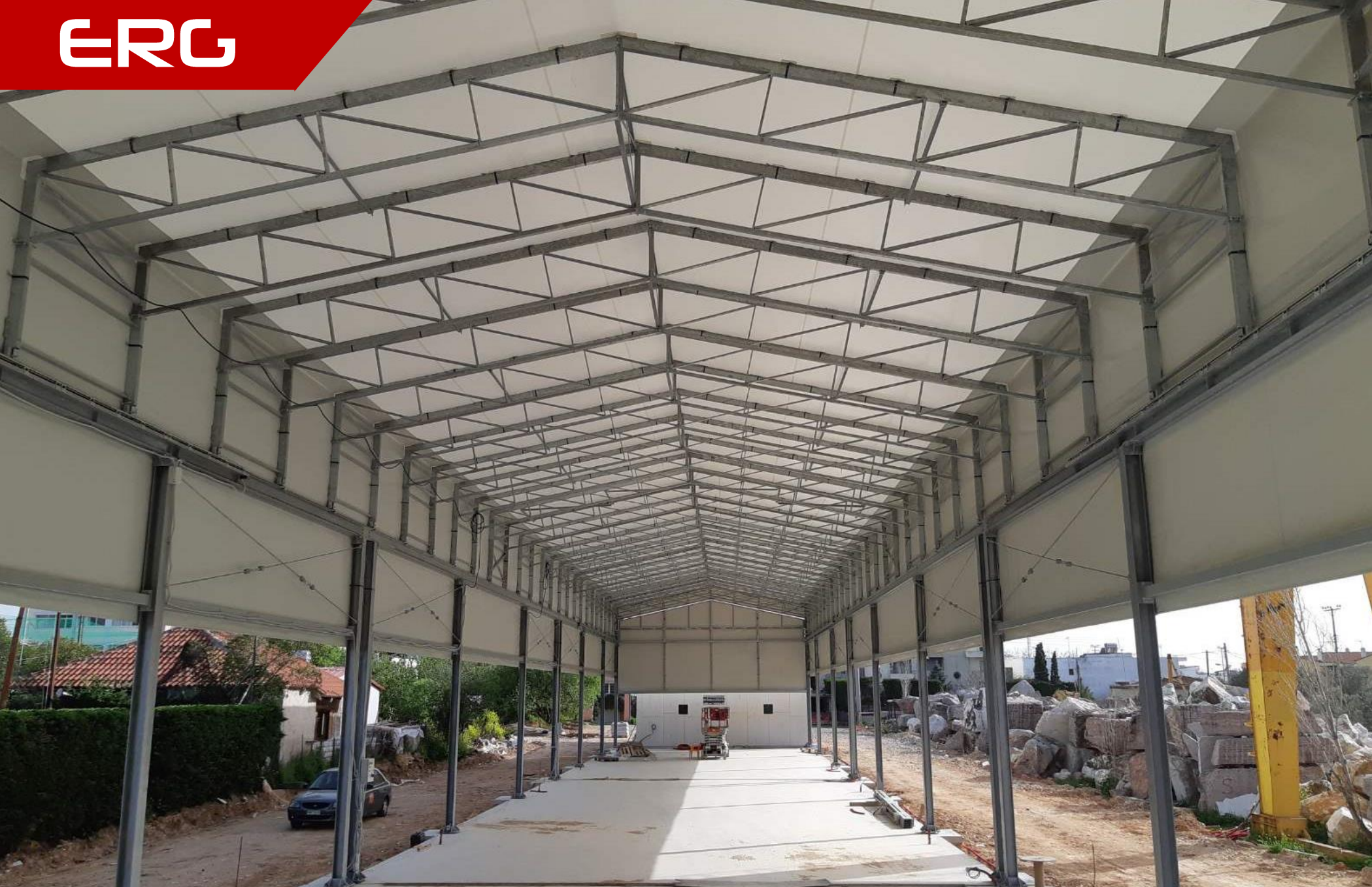
Detail of the complexity of movable roof's blocks.
