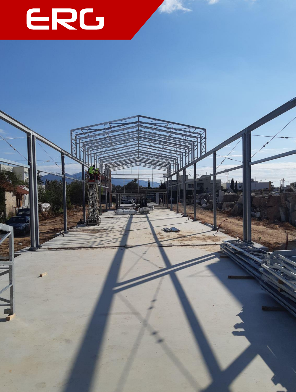
Steel structure frame with movable roof.
