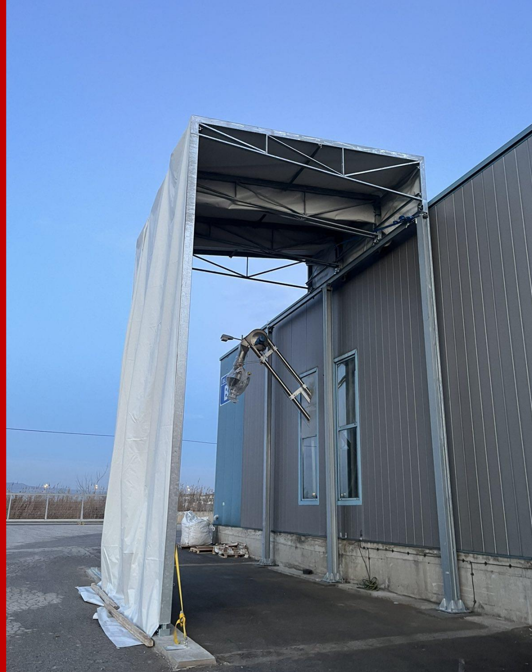
Steel structure with the PVC cover on (Under construction).
