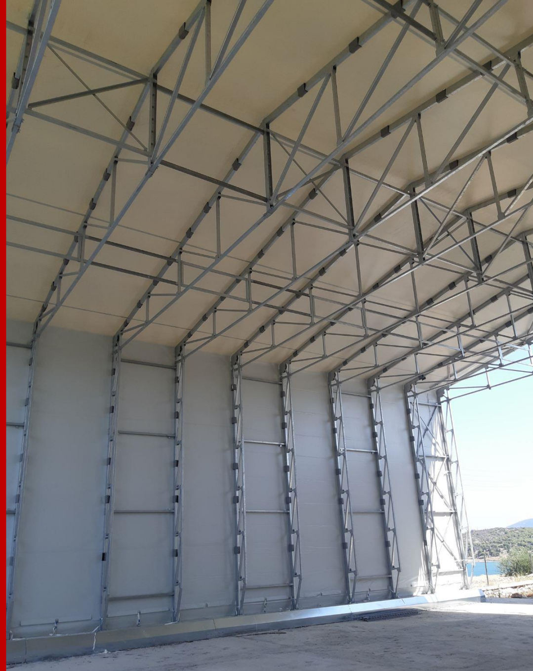
Interior of the building with view of the blocks.
