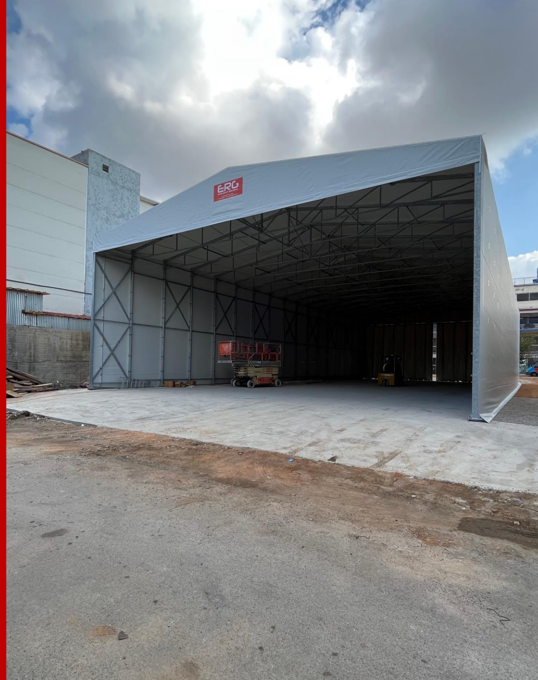
Exterior of the building with PVC cover on.
