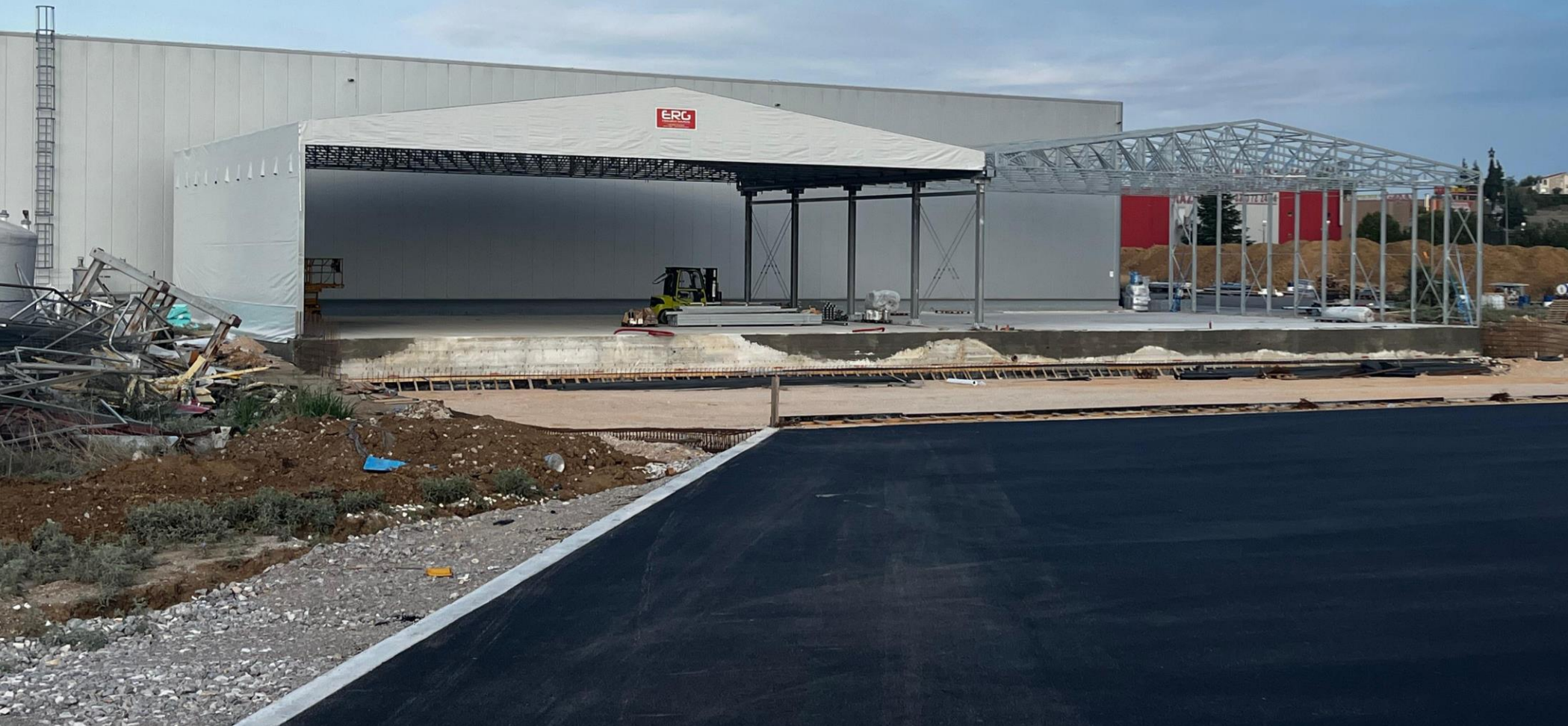
Steel structure frame (Under construction).
