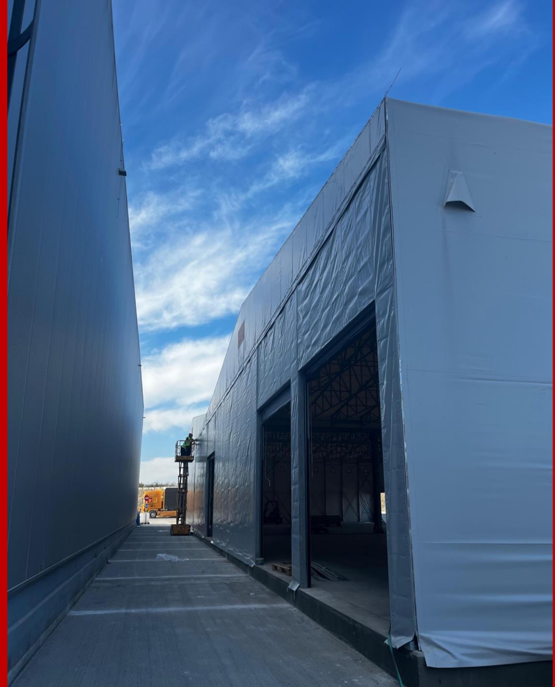
Exterior view of the buildings with PVC covers on (Under construction).
