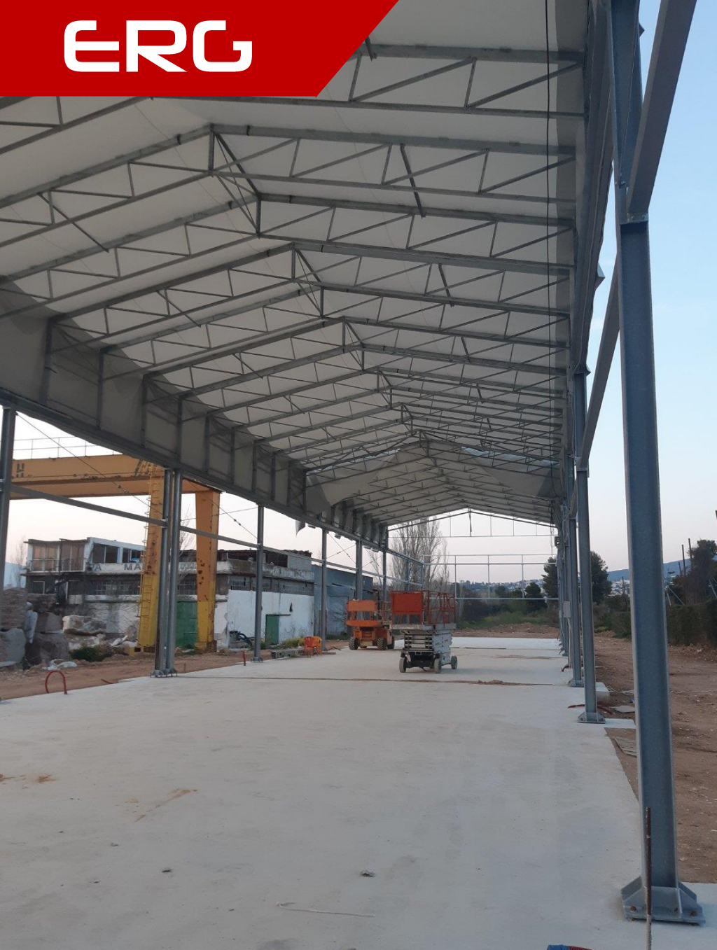
Interior of the hangar with PVC cover on. (Under construction)
