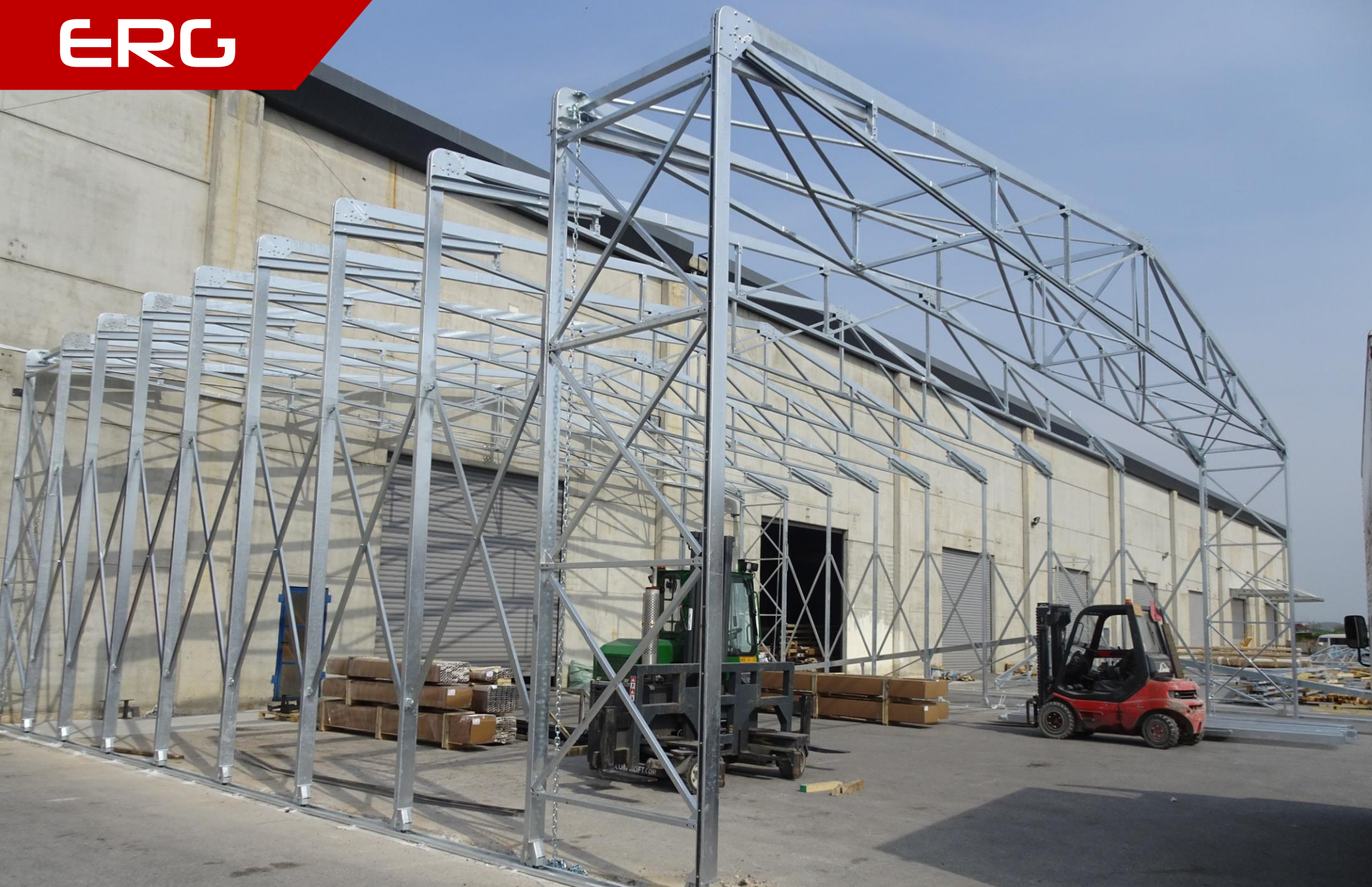
Steel structure frame.
