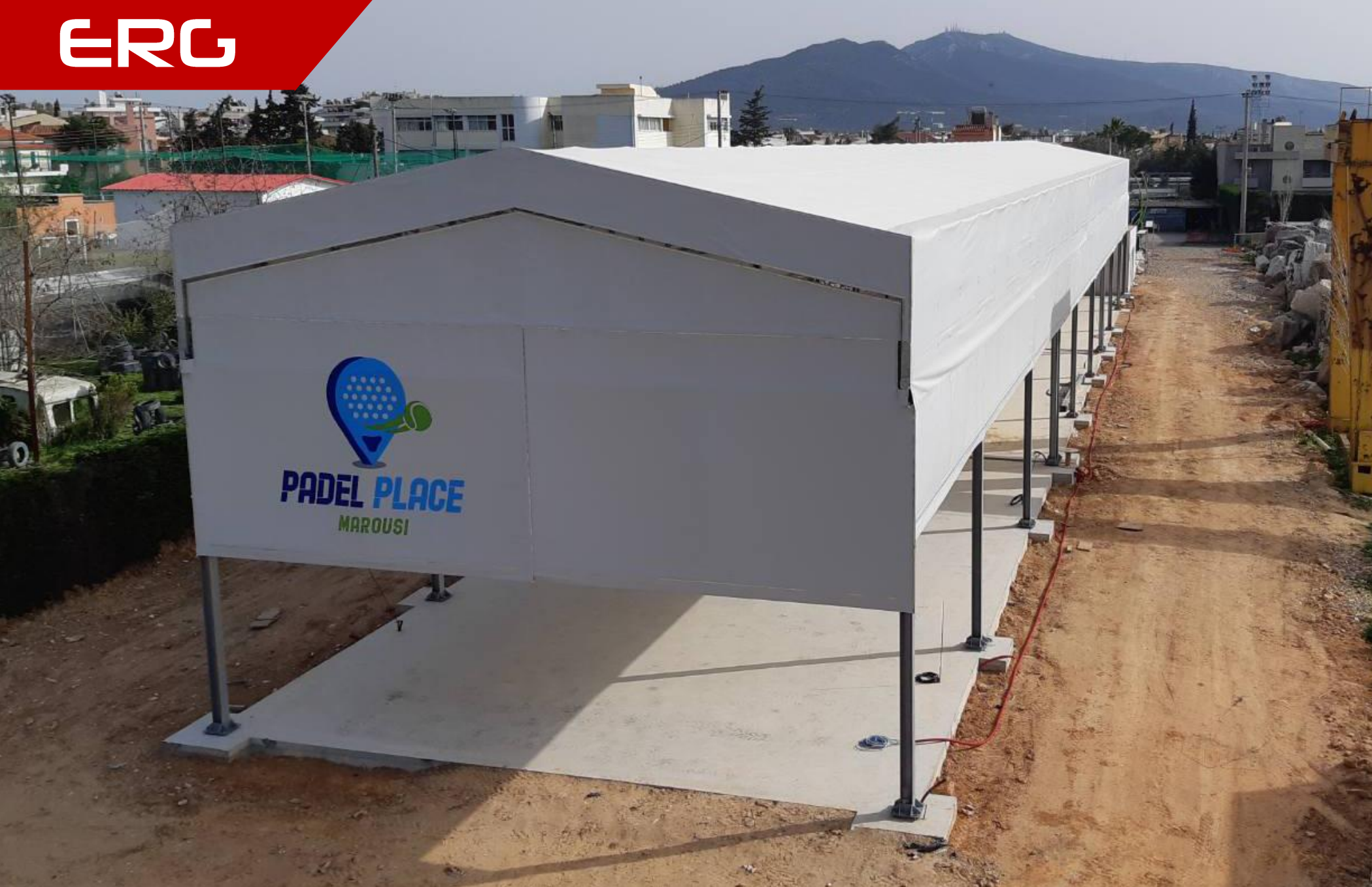
Aerial view of the entire structure.
