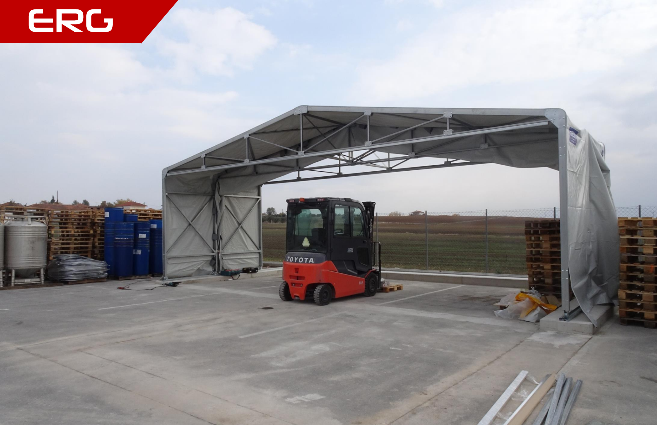
View of the building in "Closed" position. (Under construction)
