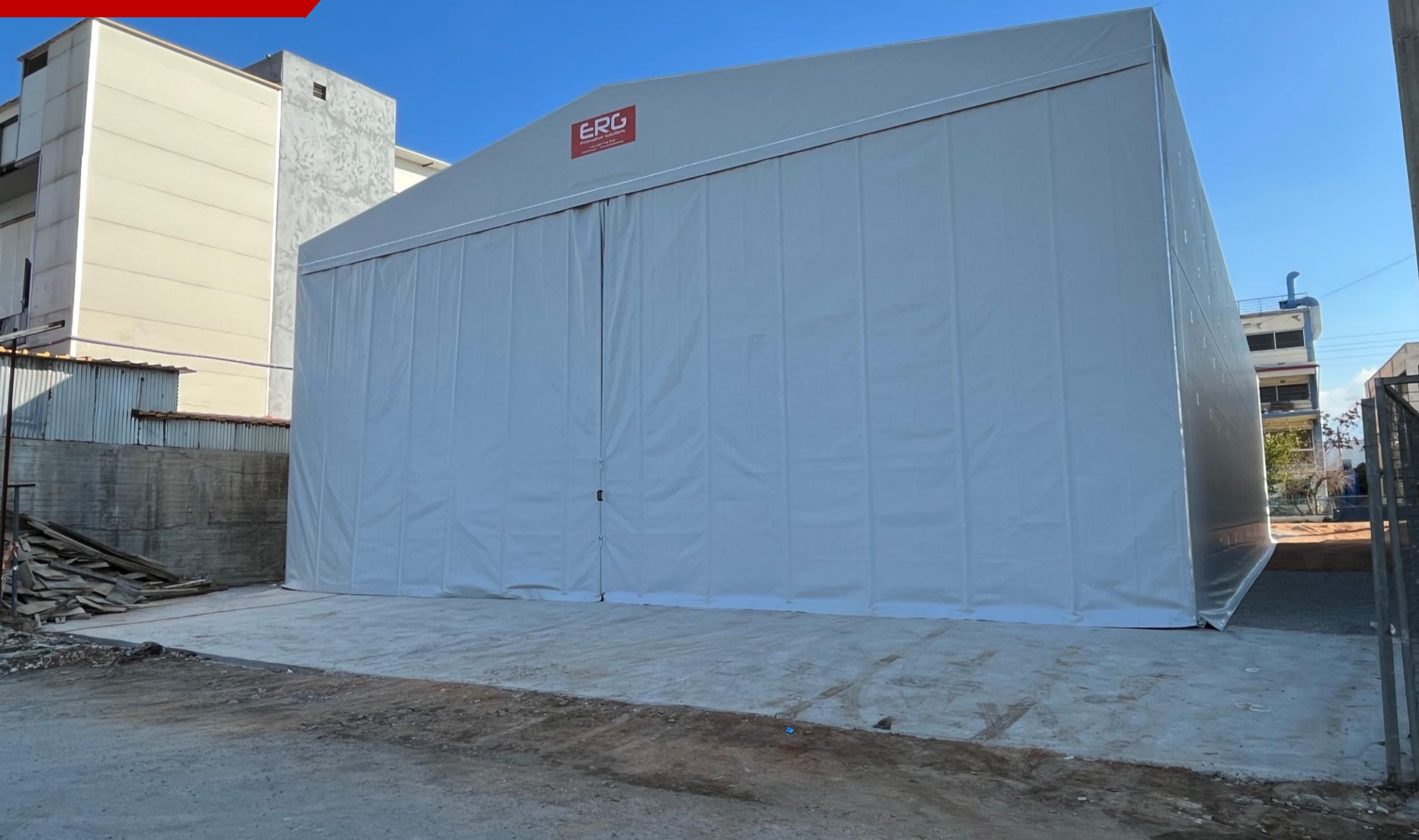
Exterior view of the entire structure.
