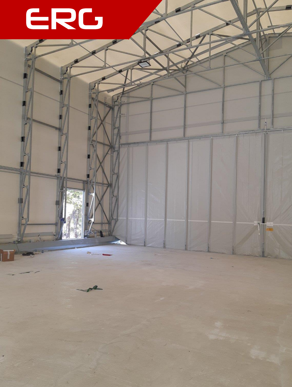
Interior of the building, with safety door.
