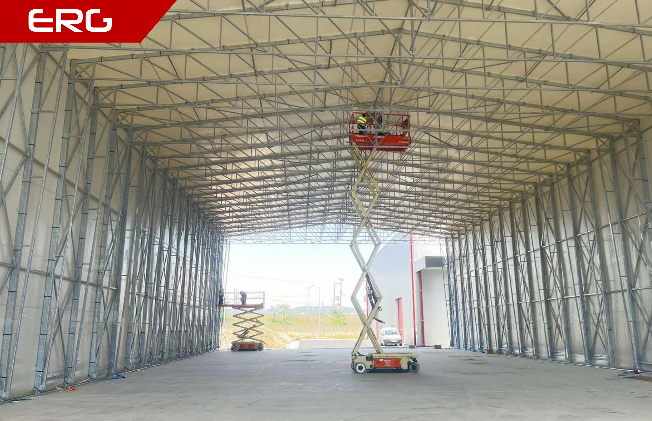
Interior view of the buildings (Under construction).
