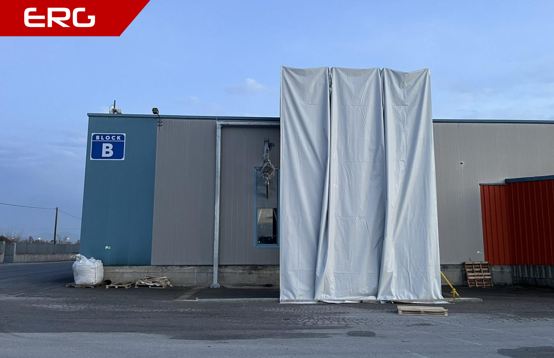
Side view of the steel structure with the PVC cover on (Under construction).
