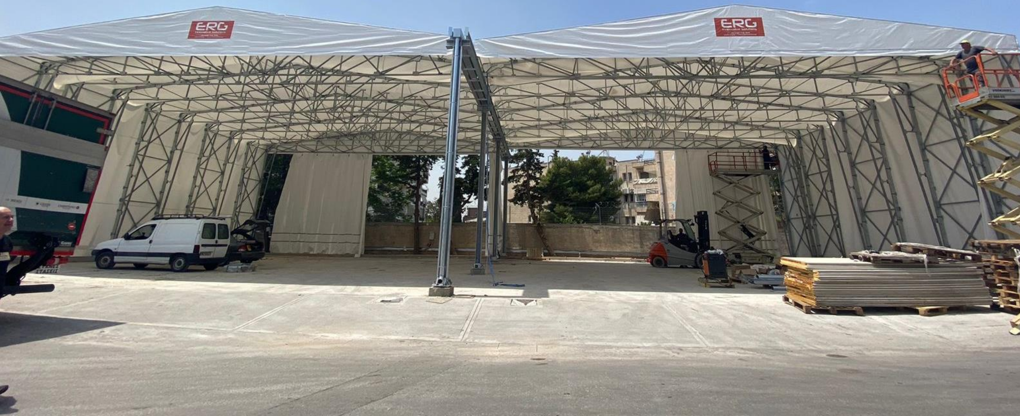
Exterior view of the double mobile building (Under construction).
