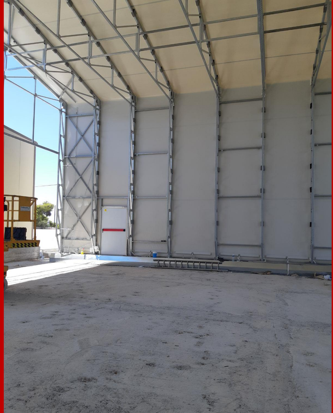
Interior of the building, with safety door.
