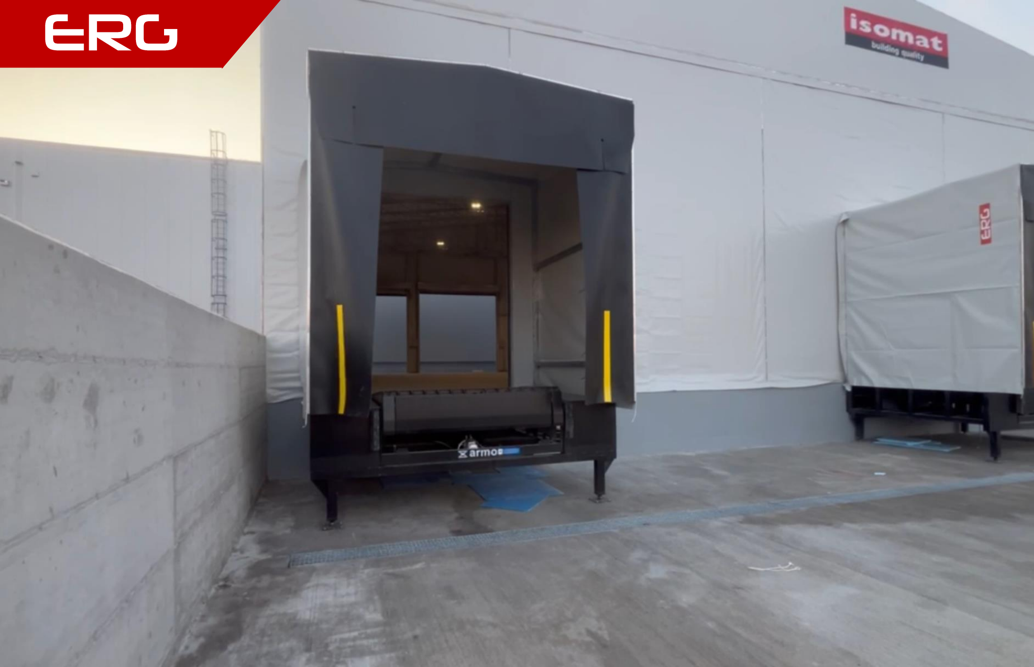
Dock shelters & ramps of the building (Under construction).
