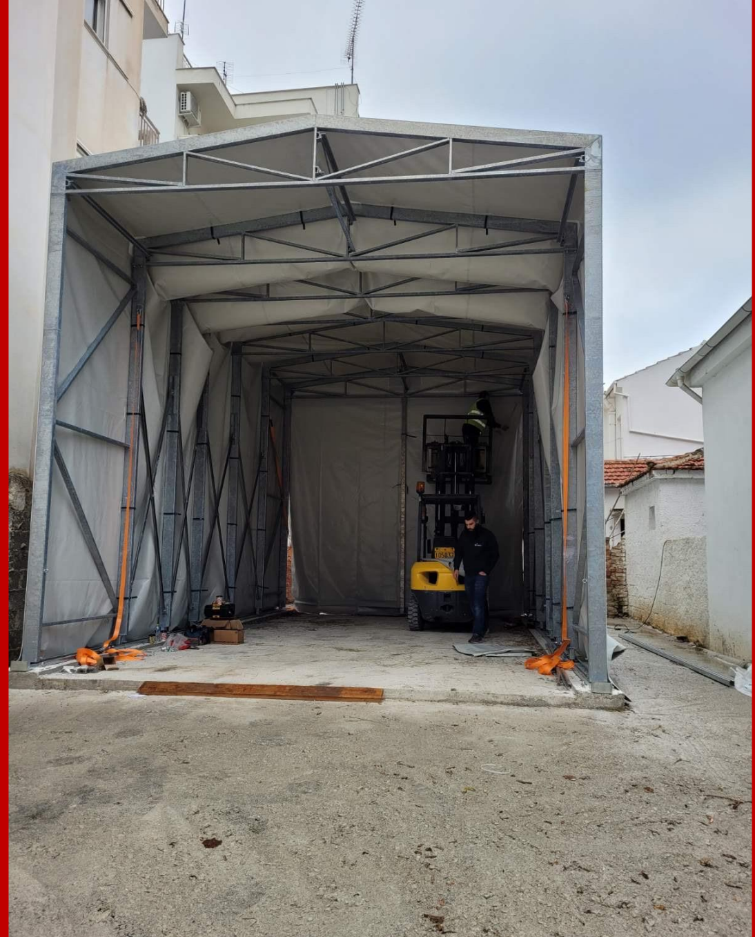
Front view of the structure.
