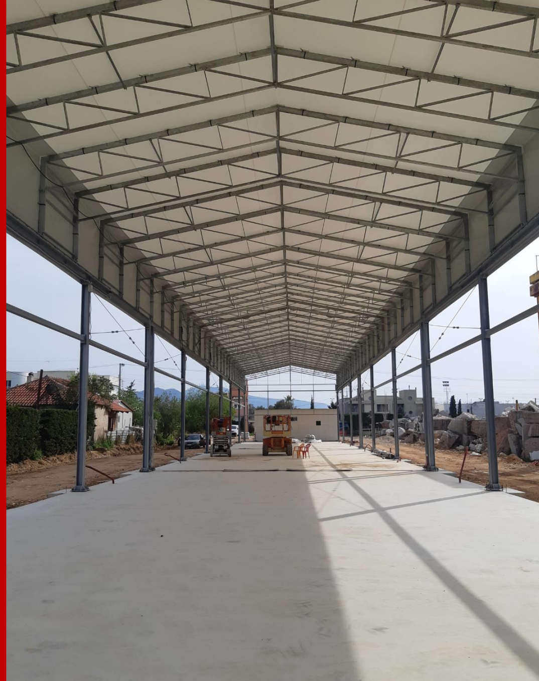
Interior of the hangar with PVC cover on.
