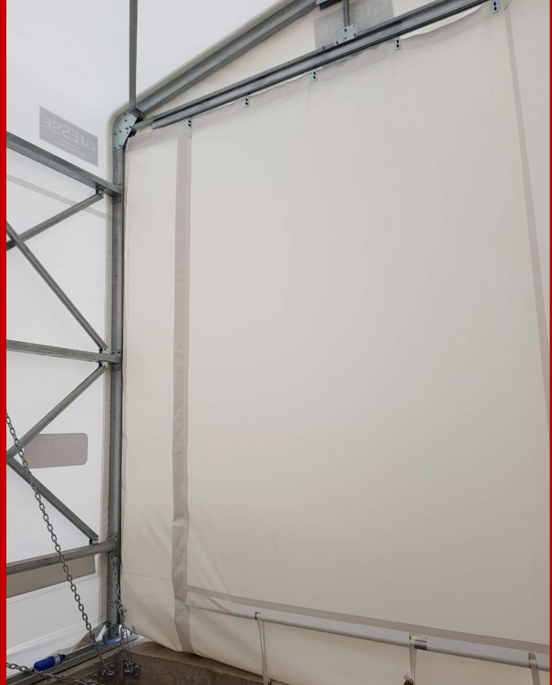
View of sliding curtain and the drive system.
