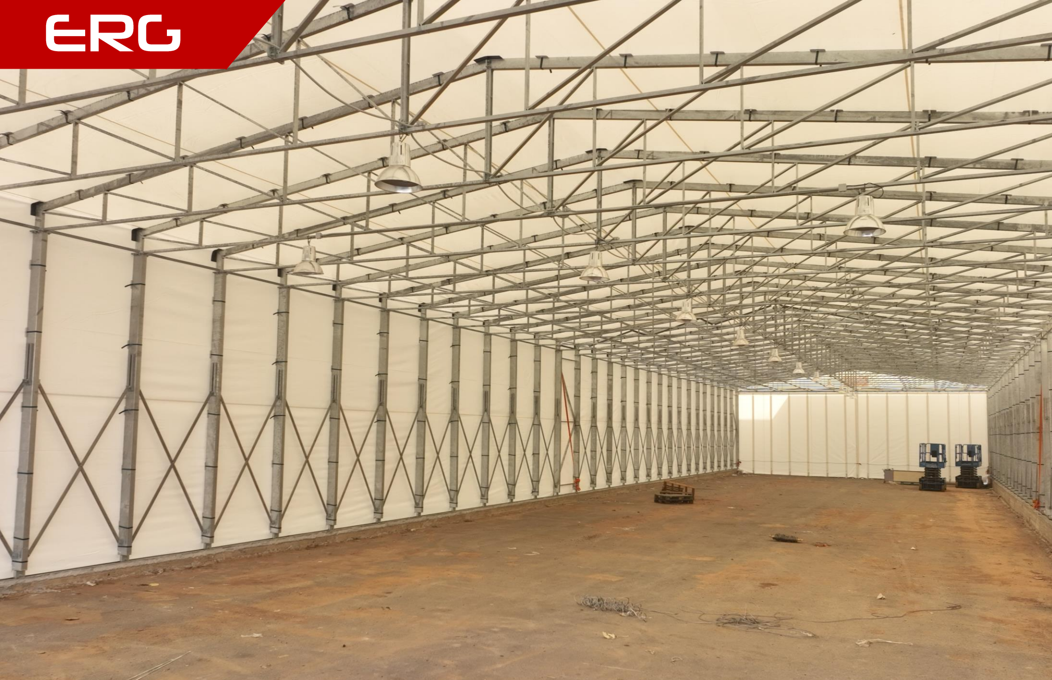
Interior of the mobile buildings.
