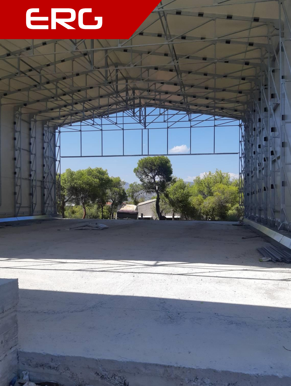
Interior of the building. (Under construction)
