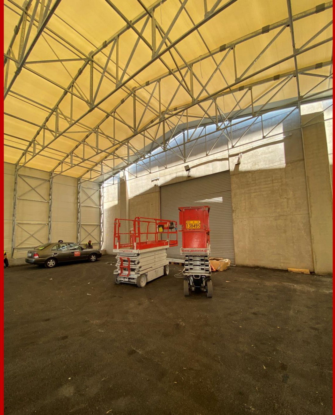
Showing of the connection with the main building.
