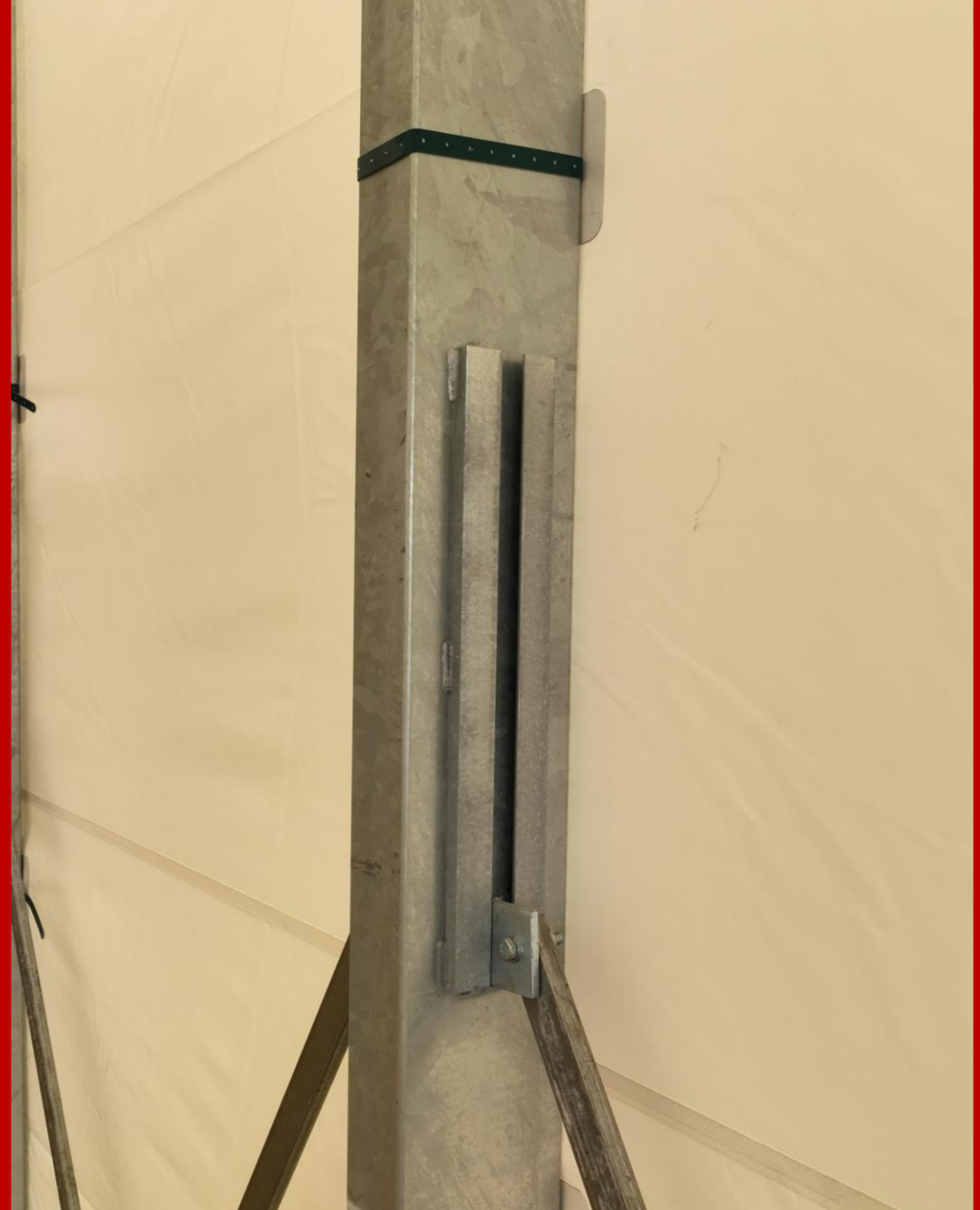
Steel structure's mobile block mechanism
