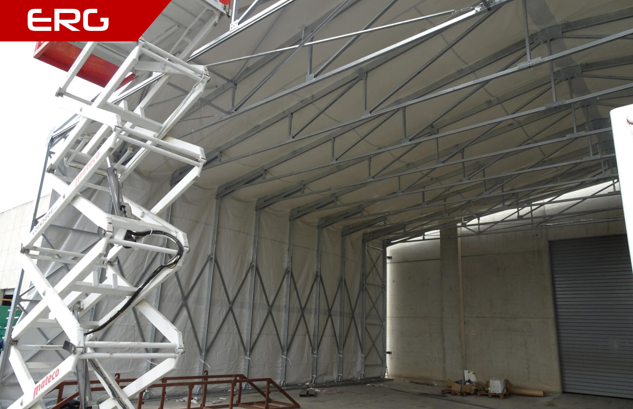
Interior of the tunnel. (Under construction)
