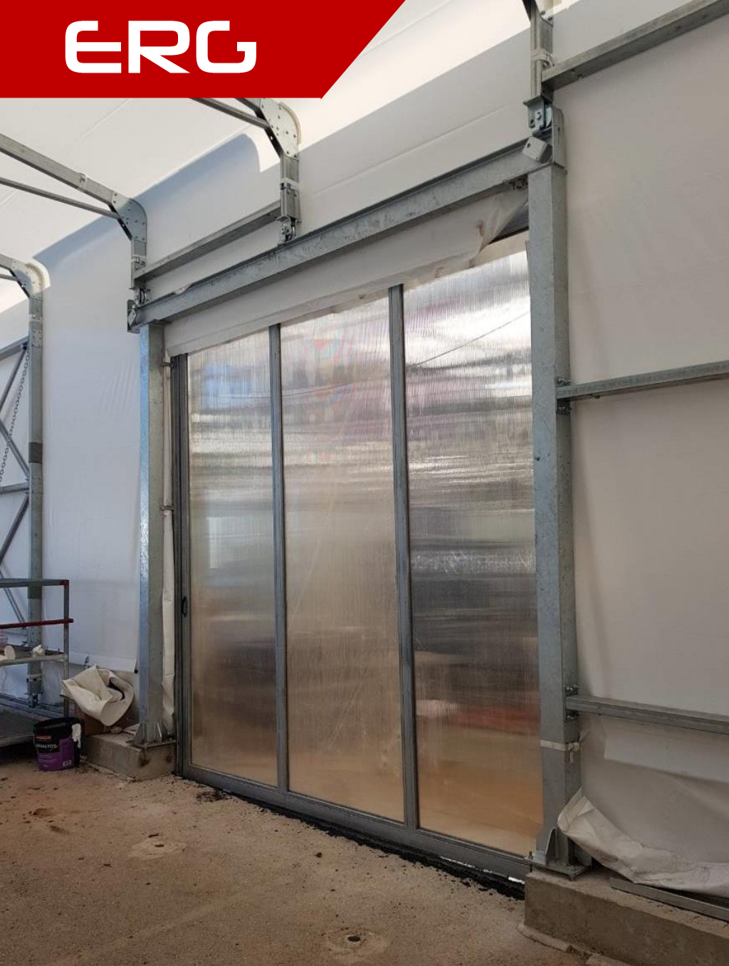
View of opening for connection with the existing building.
