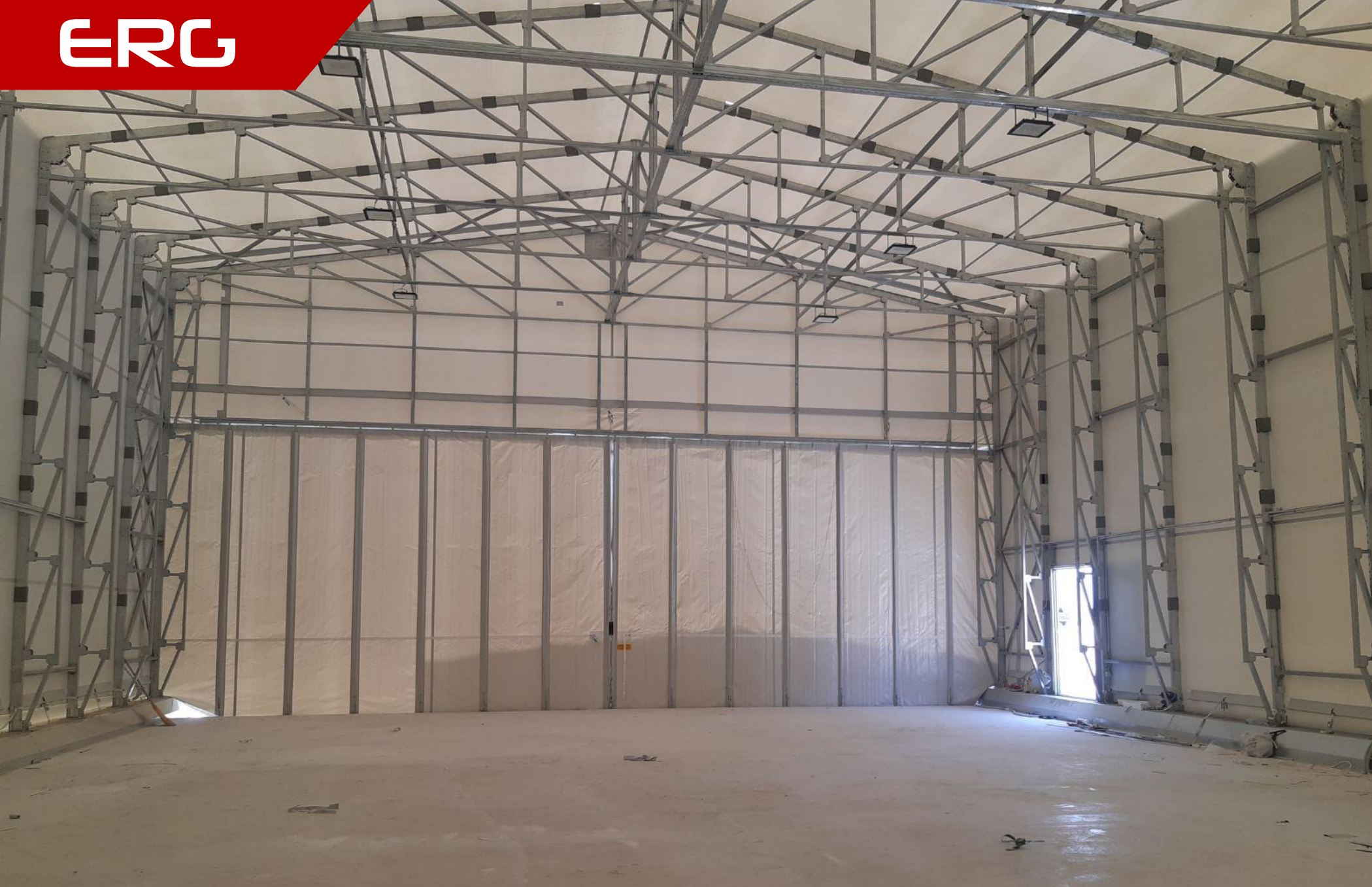
Interior of the building.
